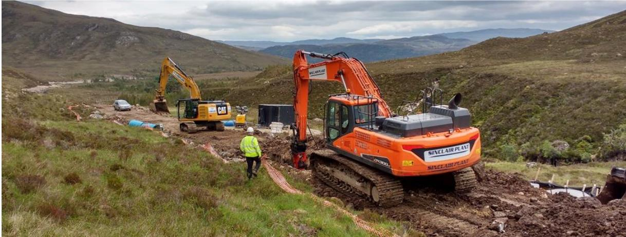
*Pictured: final stretch of penstock laying just below the intake – note the narrow working corridor.*
