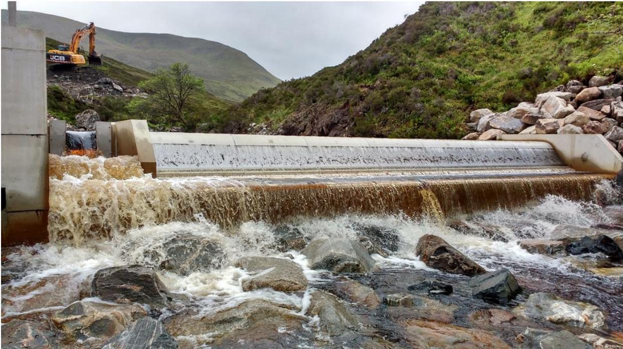
The outfall structure is complete and the screen has been installed. At the intake, work continues with grouting joints, fitting screens and the sliding penstock gate. The river bed has been reinstated to allow flows to pass over the weir (pictured) – this will allow the penstock (pipeline) to be connected to the header tank.
