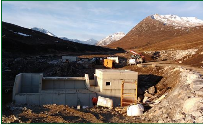
Pictured: precast units installed and made water tight.
