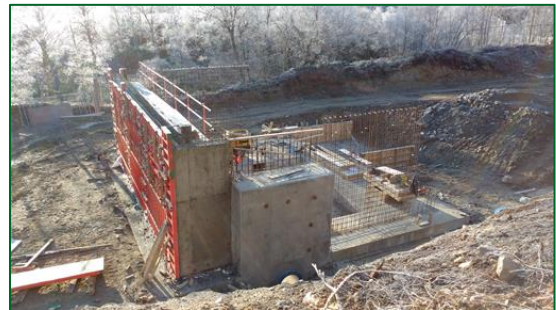
Pictured: powerhouse wall construction.
