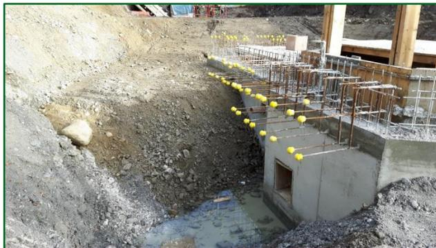
*Pictured: Alt Garbh powerhouse turbine sump cast*
