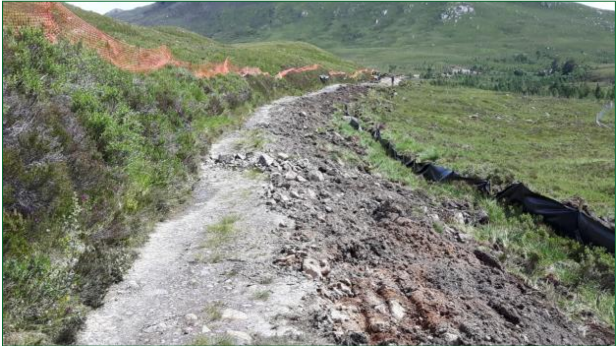
Abhainn Gleann nam Fiadh penstock corridor – turf stripping and storage.
