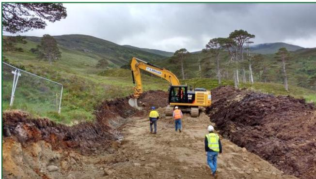
Here a temporary laydown area has been created around the site of an existing FCS borrow pit just to the west of powerhouse and all existing access road improvements have been completed, including repairing recent and historical storm damage.
